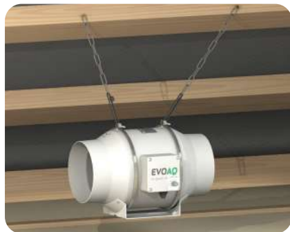
Suspend the fan with chain
